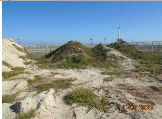
Figure 7: Topsoil stockpiles remaining on site
