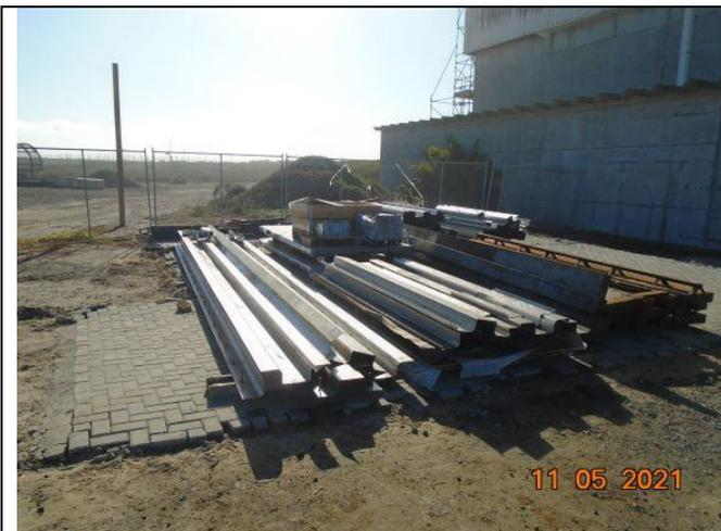
Figure 2: Stored shield panel equipment
